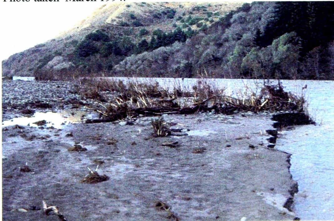
Photo 6.8. Scour beneath root zone of baffle 1 during declining storm hydrograph, 14 Jan 1995.
