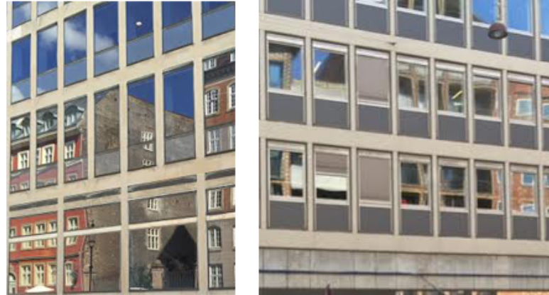
Figure 5-8: Some of the new cladding materials like metal and dark glass, that were used in the façades of office buildings built between 1960 and 1980 in Copenhagen. (To the left: located in Admiralgade 29, 1066 Copenhagen K. To the right: Located at Borgergade 28, 1300 Copenhagen K)
