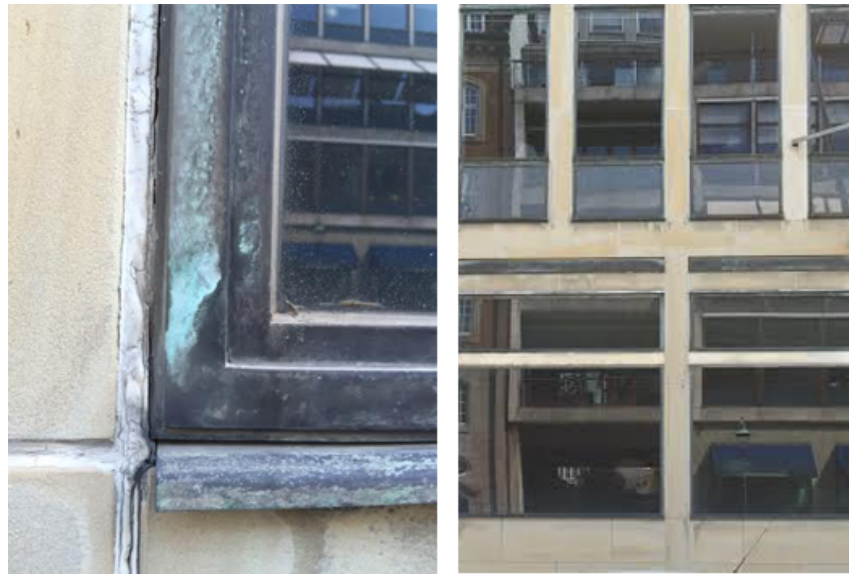
Figure 5-2: Problems in sealing materials in some parts of the façade of a Danish office building built between 1960 and 1980 (located in Admiralgade 29, 1066 Copenhagen K)
