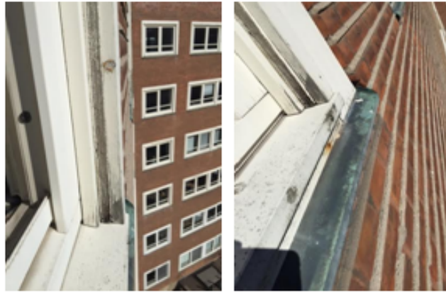
Figure 5-3: Problems in window frames which are a part of the façades of Danish office buildings built between 1960 and 1980 (Located at Dahlerupsgade 4, 1603 Copenhagen V)
