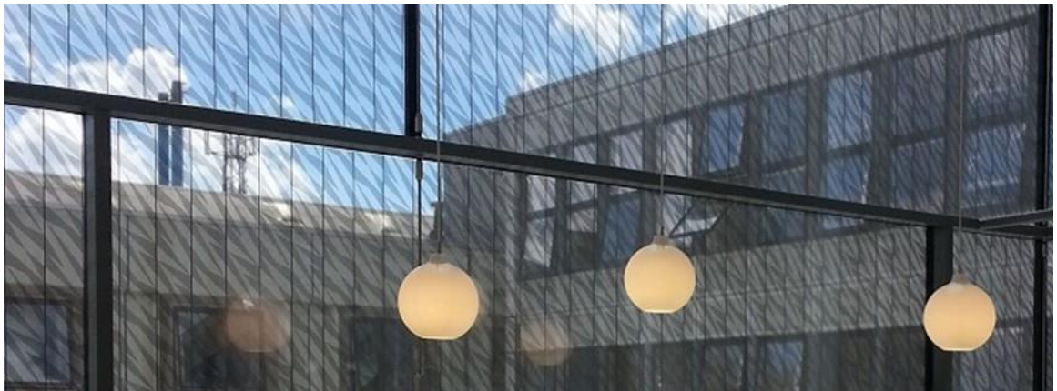
Figure 2-3 MicroShade™ is a new generation of modern, energy efficient façade and roof glazing as an alternative to the conventional solar shading solution for new and refurbished buildings
