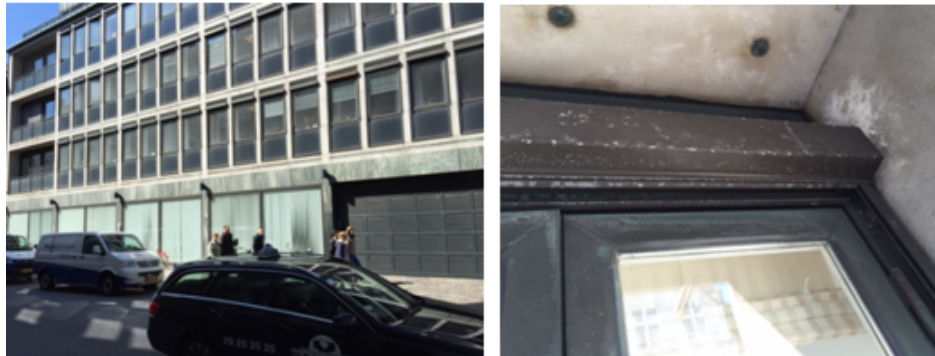
Figure 5-4: Problems and corrosion in metal frames of window which are part of the façade of a Danish office building built between 1960 and 1980 (Located at Bredgade 43, 1260 Copenhagen K)
