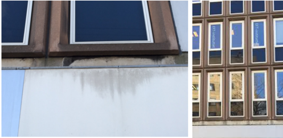
Figure 5-1 Problems like mould in the façade of a Danish office building built between 1960 and 1980 (Located at Borgergade 28, 1300 Copenhagen K)
