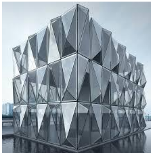
Figure 5-27 The Schüco Parametric System, with a geometrically freeform 3D façade design.
