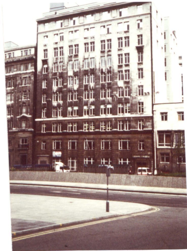
Figure 4.15 The soiling pattern which emerged after four years of the building being cleaned, located in Dock Road, Liverpool.
