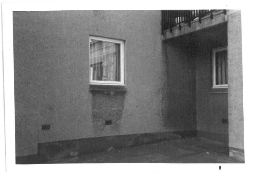
Figure 4.17(a) An example of dirt washing on a 17-year old Edinburgh housing estate
