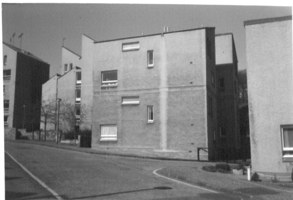
Figure 4.17(b) An example of white-washing (by the action of a leaky pipe) on a 17-year old Edinburgh housing estate
